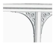
Image shows gallows brackets fitted to gutter channel and post.
